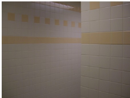
Figure 2: No "line of sight" issues in women's restroom
