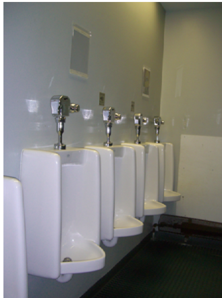
Figure 2: Urinals in men's restroom
