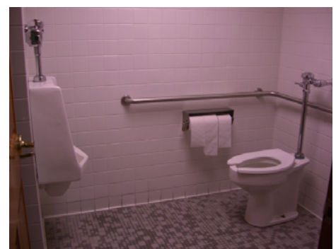
Figure 4: Unisex restroom outfitted with toilet and urinal - no changing station.
