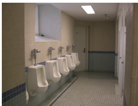
Figure 7: Men's Restroom - No partitions between urinals.
