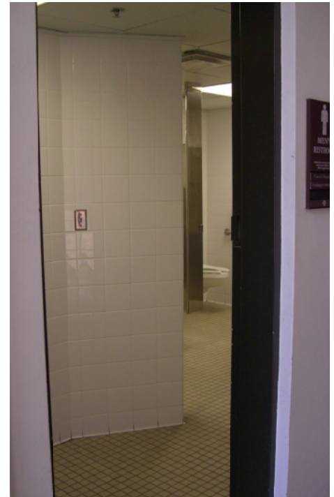
Figure 2: Line of site issue from the hallway into the universal design stall in the men's restroom on the main lobby level.
