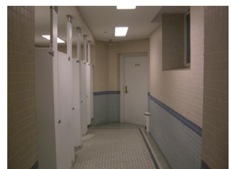
Figure 8: Women's Restroom partitions are too close together and the distance from the ground is too high.
