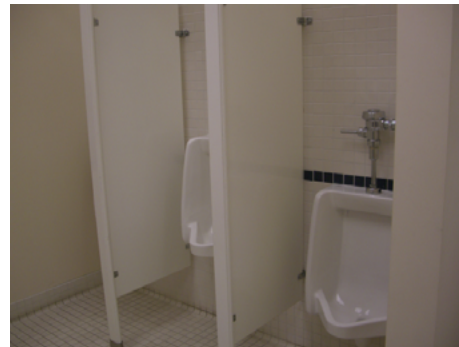
Figure 2: Men's restroom partitions are present, deep, and have adequate spacing.
