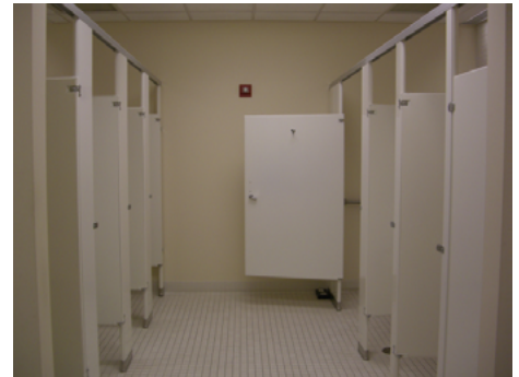
Figure 4: Women's restroom partition distance from the ground is too high. There is an adequate number of partitions for the size and function of the facility and they are well spaced.
