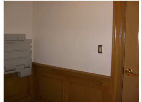
Figure 2: Baby-changing station in first floor women's restroom.
