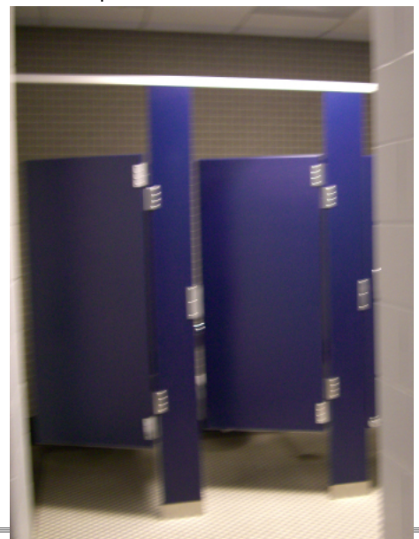
Figure 6: Bathroom stalls in the Women's Restroom on entrance level.
